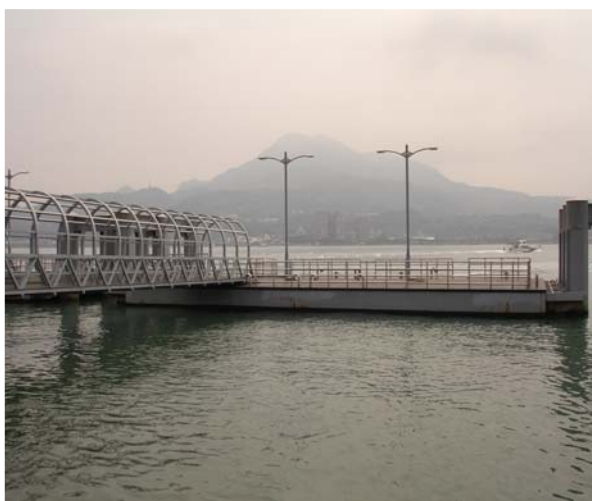
照片 9, 鋼板製浮箱 (22M*8M*1.5M)
